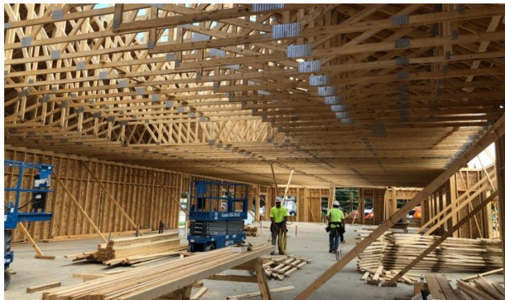
North Building Interior
