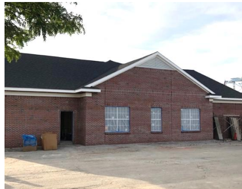
Back of the Expansion
