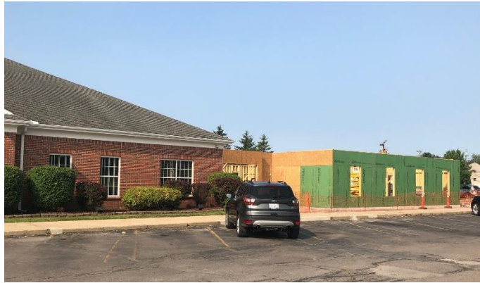
Expansion of Main Office
