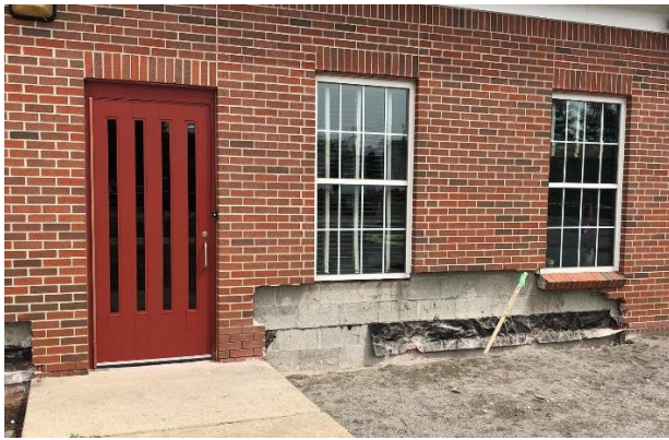
Back of Building
