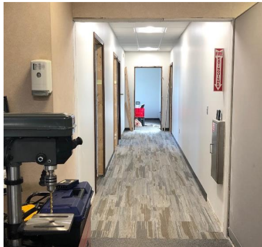
Newly Renovated Hallway
